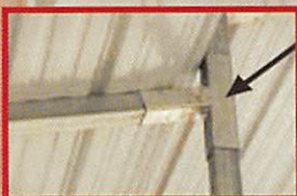
Stronger construction (barns with welded supports)
